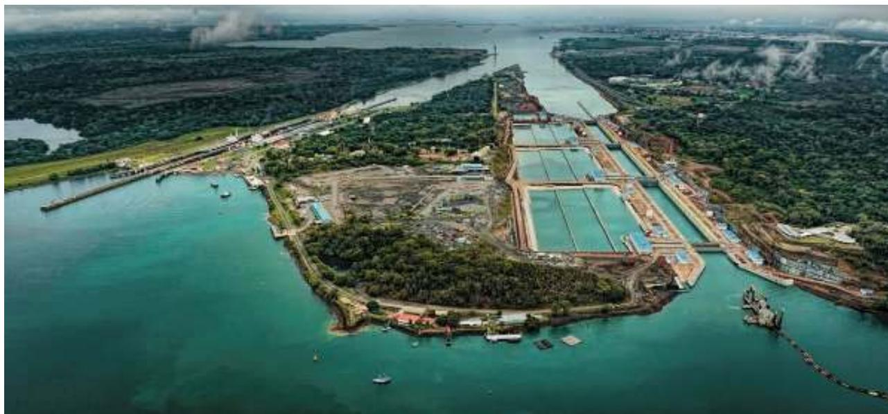
Above is an aerial photograph of a set of the new expanded locks in the Panama Canal on the right. On the left are the original locks. Besides allowing the passage of larger vessels (13-14,000 TEUs [twenty-foot equivalent units] v. 5,000 TEUs), the new locks use the three reservoirs to the side of each lock to recycle 60% of the water per transit, for a much more efficient use of this resource.
